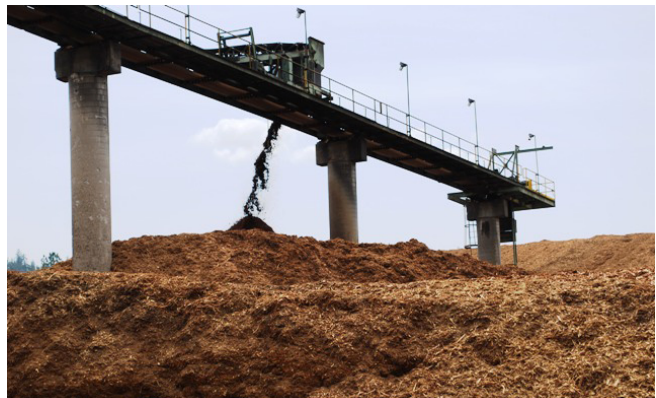
Woody biomass processing facility.
